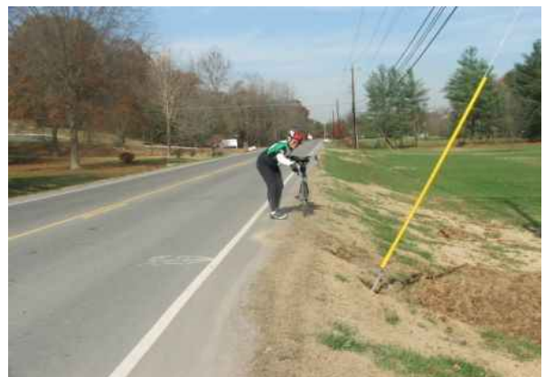
Illustration 6: Section of New Shackle Island Road/258 where nature is reclaiming shoulder.
