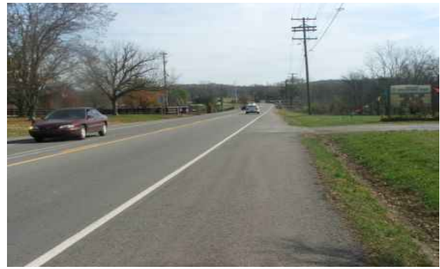
Illustration 4: Approach to bridge over Station Camp Creek. No shoulder over bridge.
