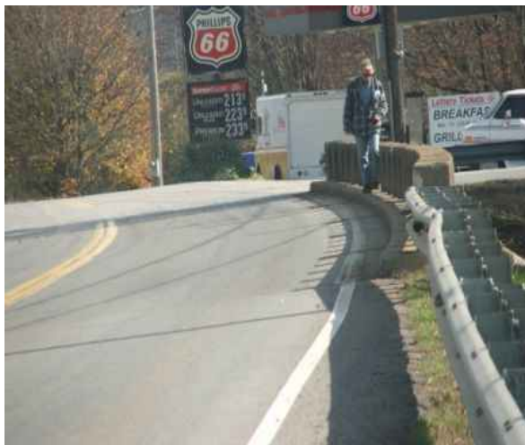
Illustration 5: Close up of bridge across Station Camp Creek.
